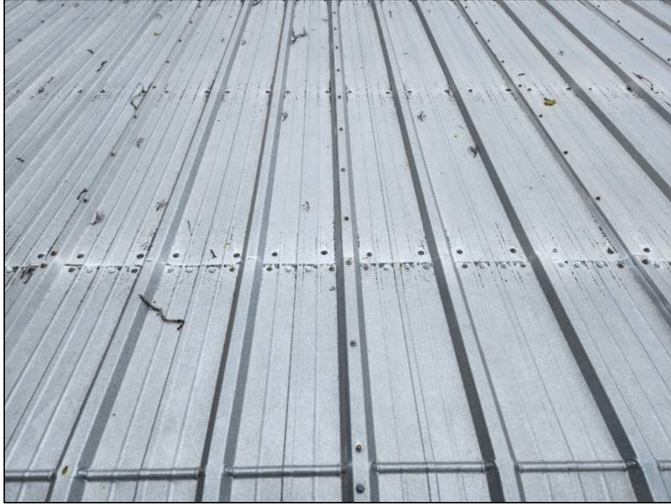
Roofing and Fasteners.
