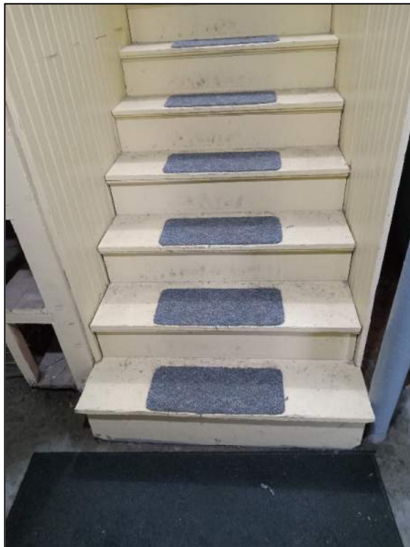
Worn Treads and Nosing on Wood Stair to Basement.
