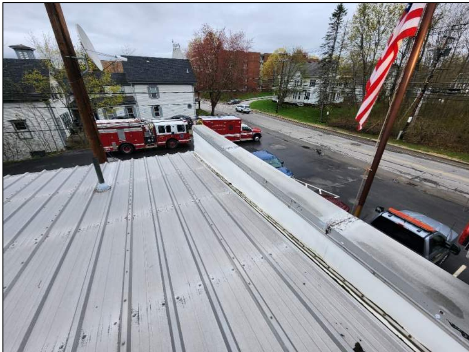
Termination Bar at Parapet Wall.
