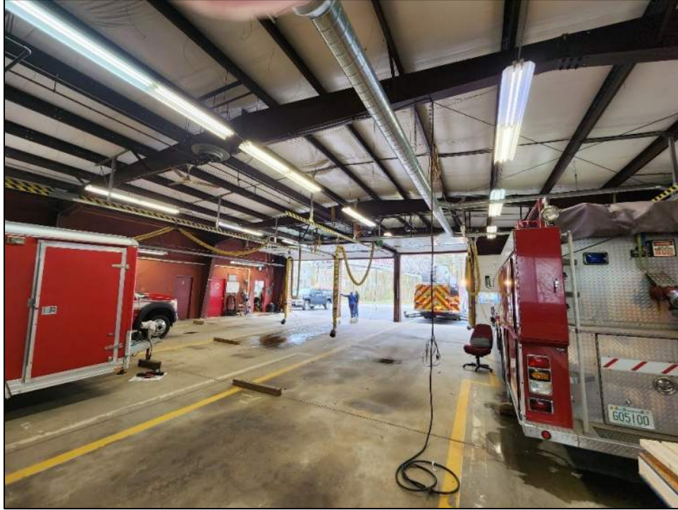
Pre-Engineered Bent and Roof Purlins.
