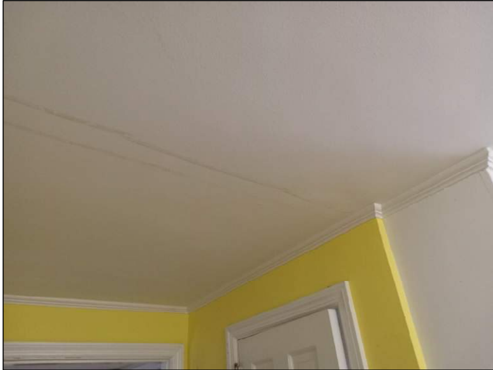
Patched Ceiling in Residence Kitchen from Removed Wall.
