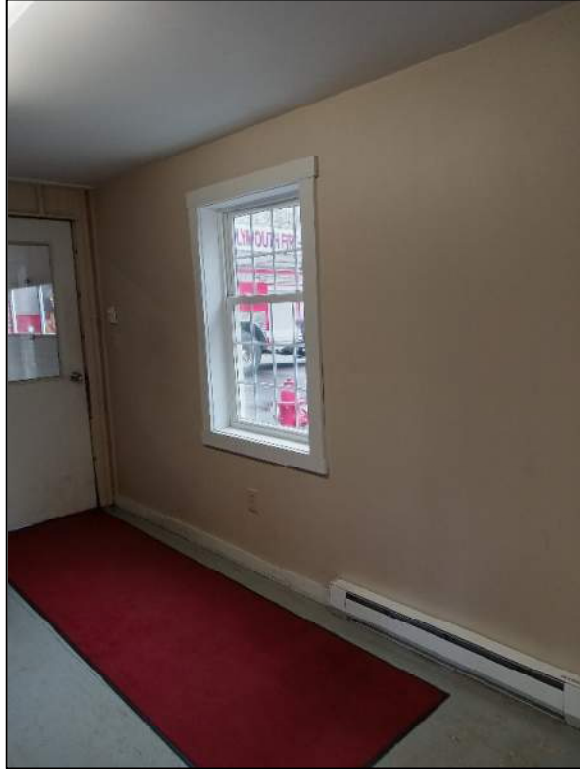
Non-Fire-Rated Wall Assembly Between Apparatus Bay and Addition to Residence.
