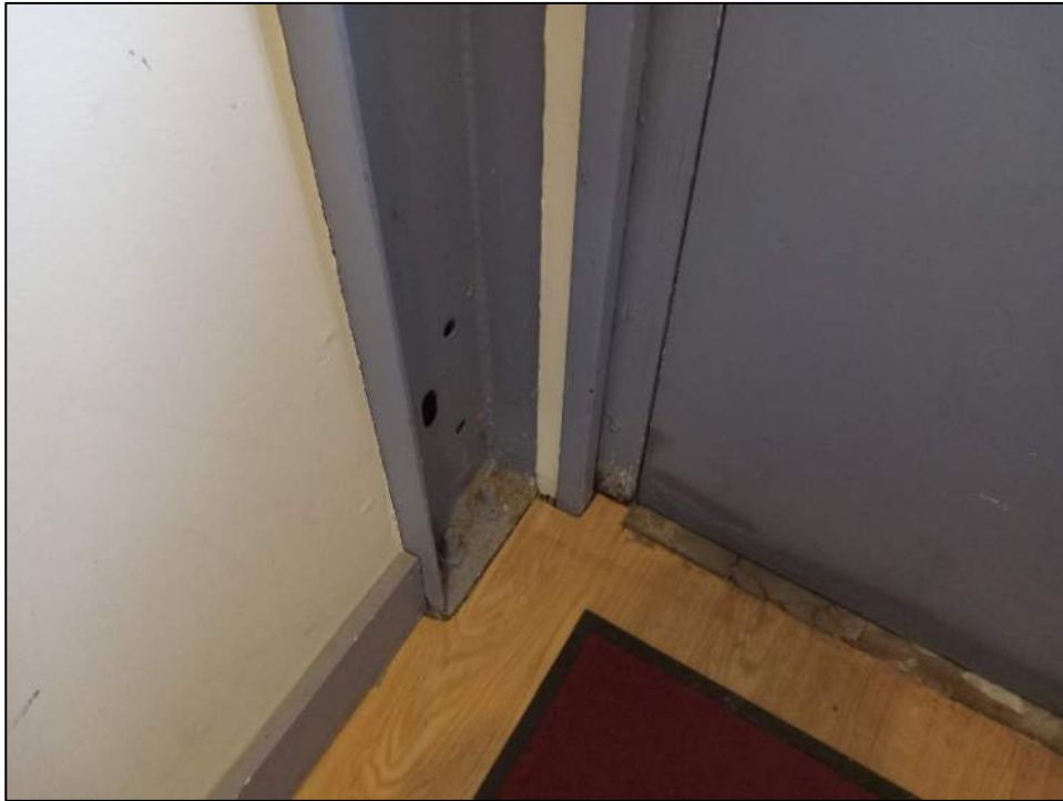
Rusted Exterior Door in Original Metal Building and Exposed Concrete.
