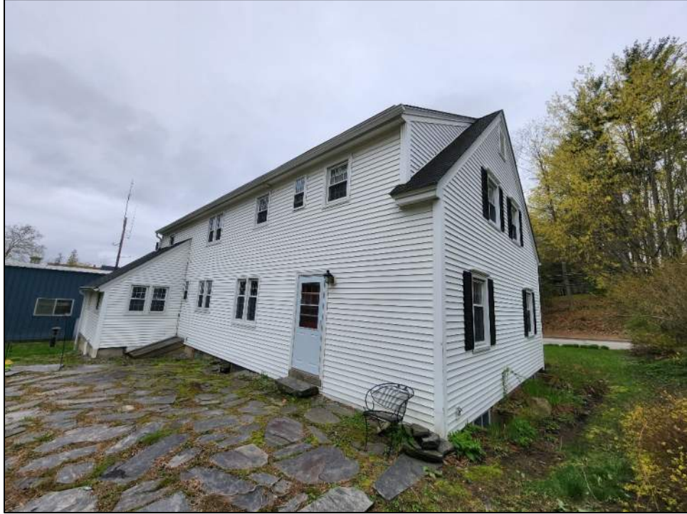
Office Rear - North and West Side.
