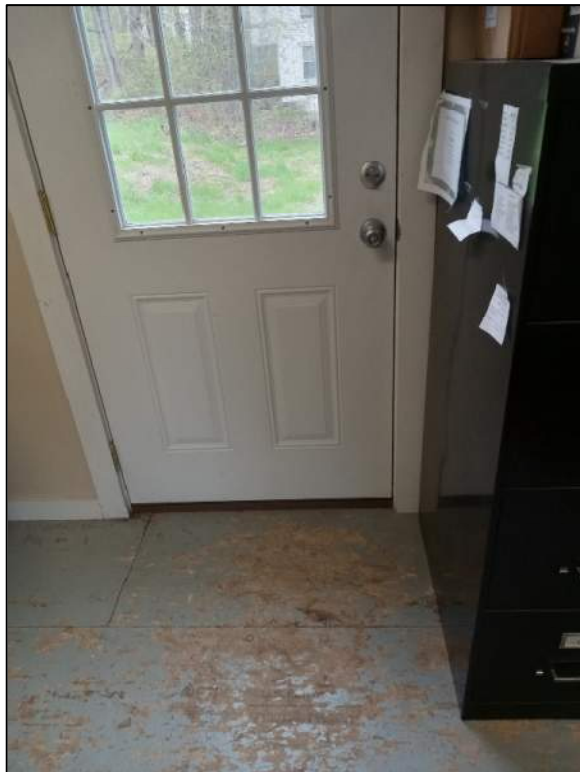
Worn Painted Plywood Flooring.
