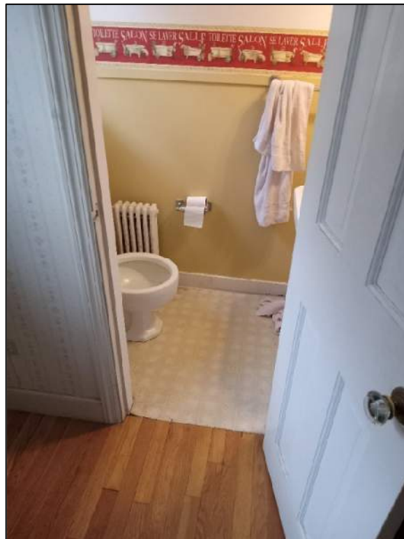
Transition Strip Between Dissimilar Floor Finish Surfaces.
