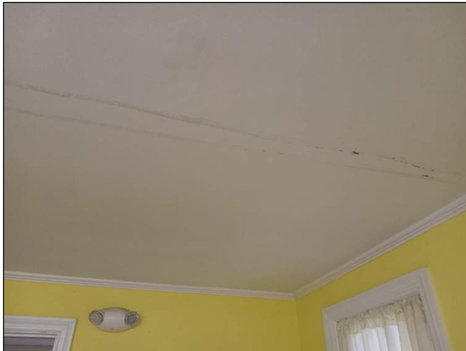
Patched Ceiling in Residence Kitchen from Removed Wall.
