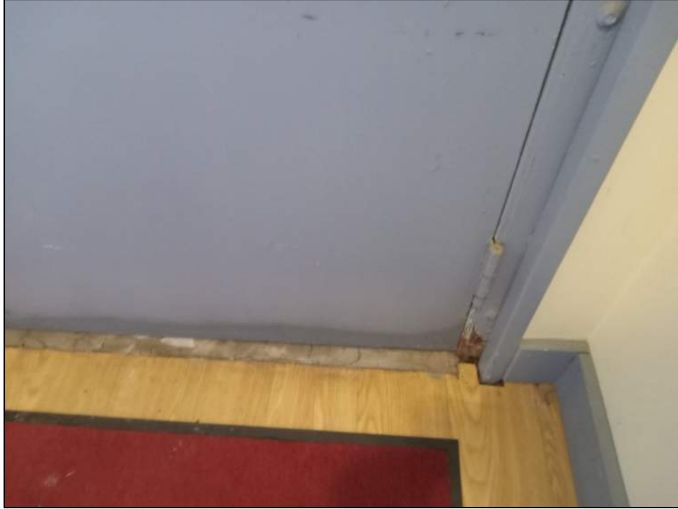
Rusted Exterior Door in Original Metal Building and Exposed Concrete.
