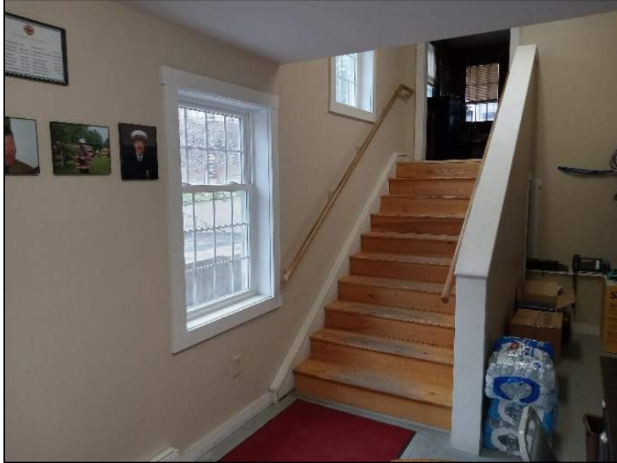
Worn Stained Wood Stair Treads and Nosing.
