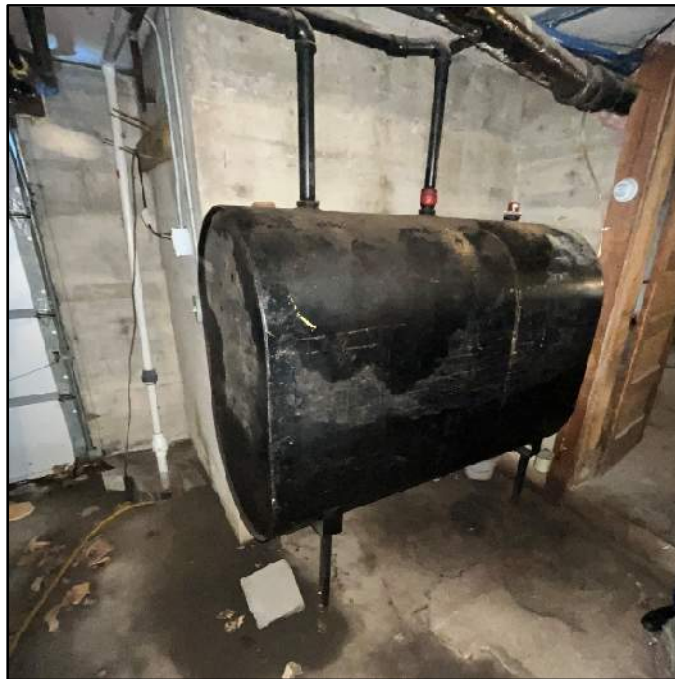
The existing oil tank in the basement of the residence house.
