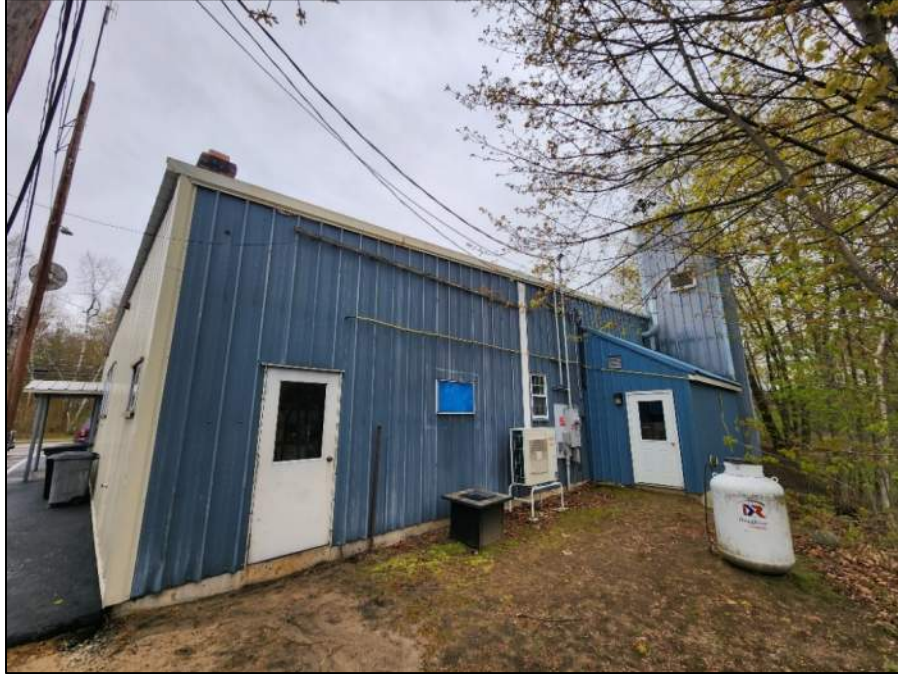
Former In-filled Exercise Room Window.
