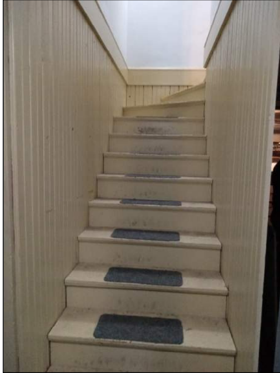
Worn Treads and Nosing on Wood Stair to Basement.
