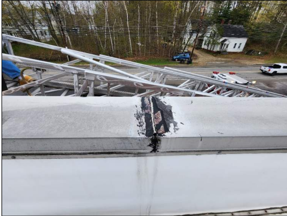
Sealant Joint at Top of Parapet Wall.
