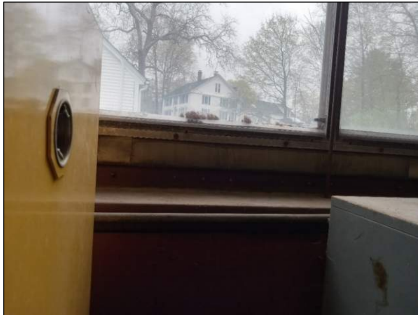
Single Glazed Metal Windows in Apparatus Bay.
